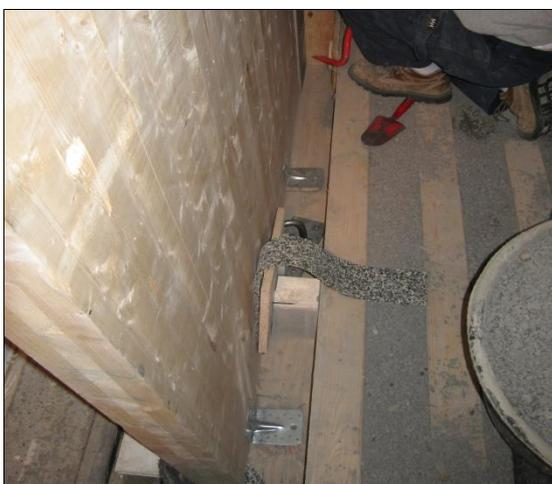
Figure a: T-junction with cross laminated timber (RE GT Wal)
