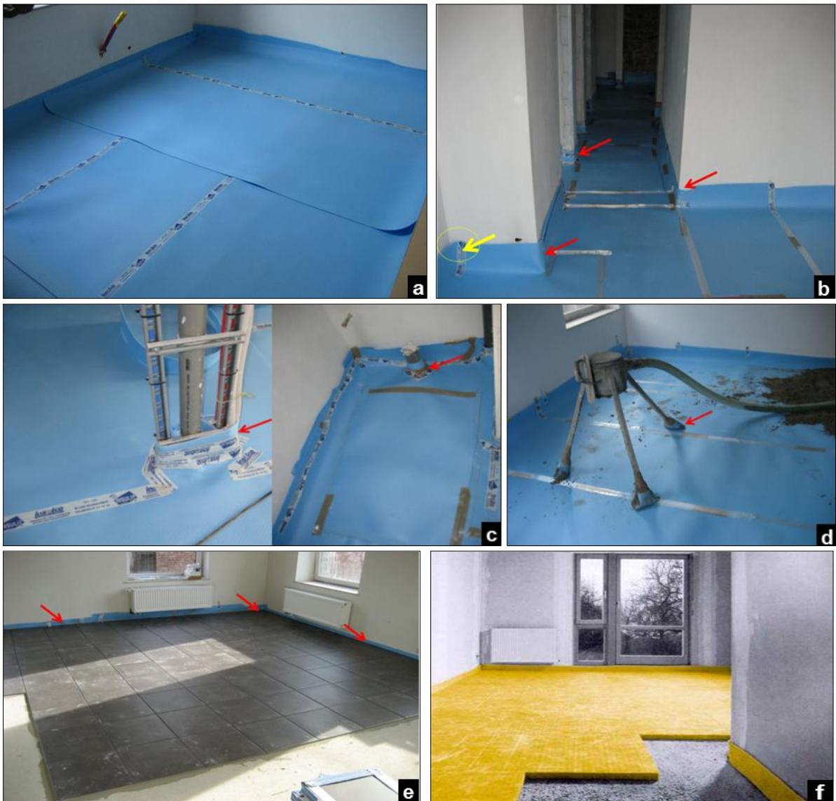
*Figure34: the correct placing of the floating floor is vital. Even small hard contacts will eliminate all positive effects! If a material with open cells is used as an elastic interlayer (e.g. mineral wool, see right picture), a plastic foil should be applied before installing the screed.*
