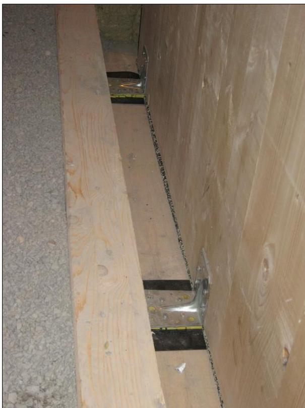
**Floor 'd'** cross laminated timber 9.4 cm thick, with wooden 'ribs' (see drawing) of 9.5x20 cm<sup>2</sup>, interdistance 25 cm. The space between the 'ribs' is filled with gravel (1400 kg/m<sup>3</sup>).
