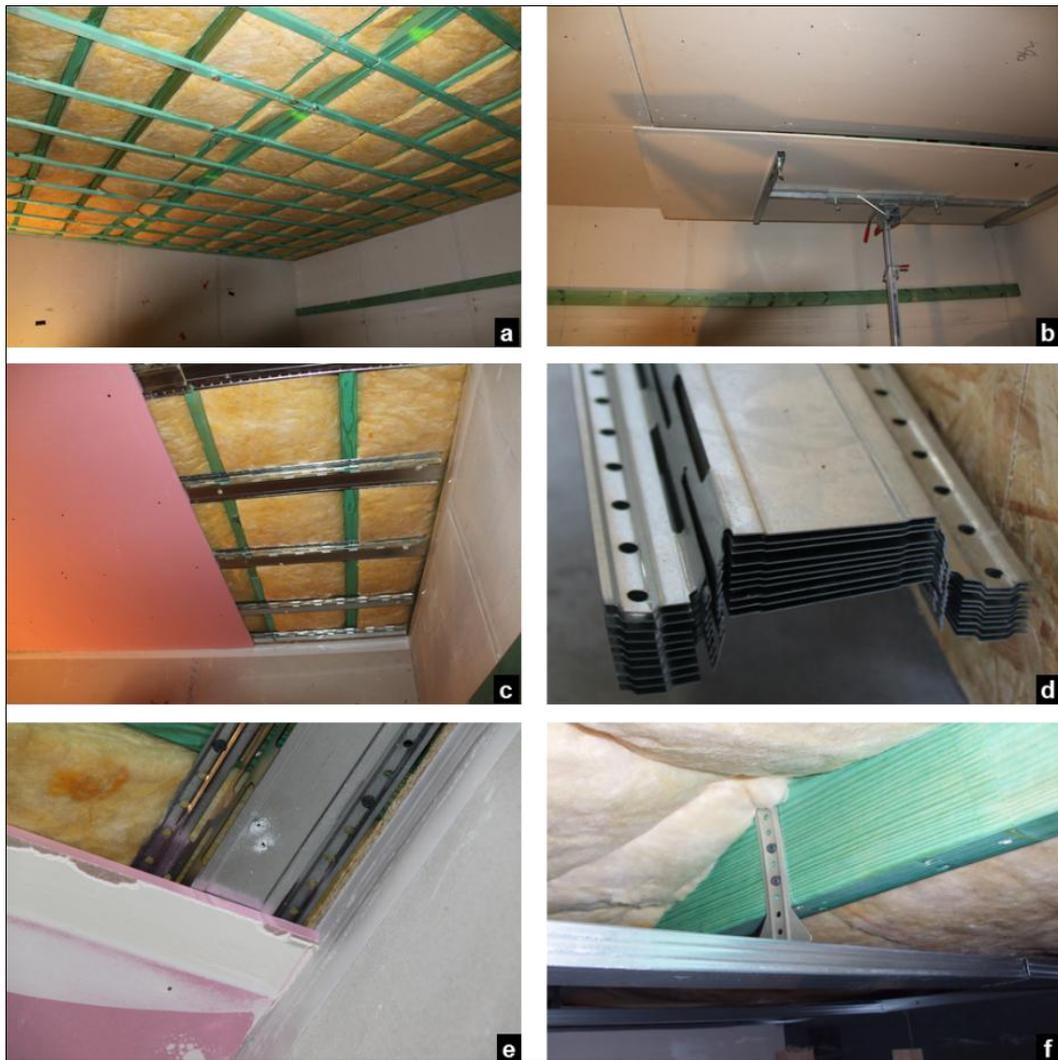
Figure 40: (a) Wood furring strips fixed directly and perpendicular to the joists of the floor, this is only suitable for floors within the same building. (b) Mounting device to fix any heavy boards (c) (d) Ceiling metal profiles (Knauf) allowing a resilient connection with the joists (e) The finishing of the joint between wall and ceiling has an influence on the direct and flanking insulation. (f) Another type of fixation of metal ceiling profiles allowing for a larger cavity (Gyproc).
