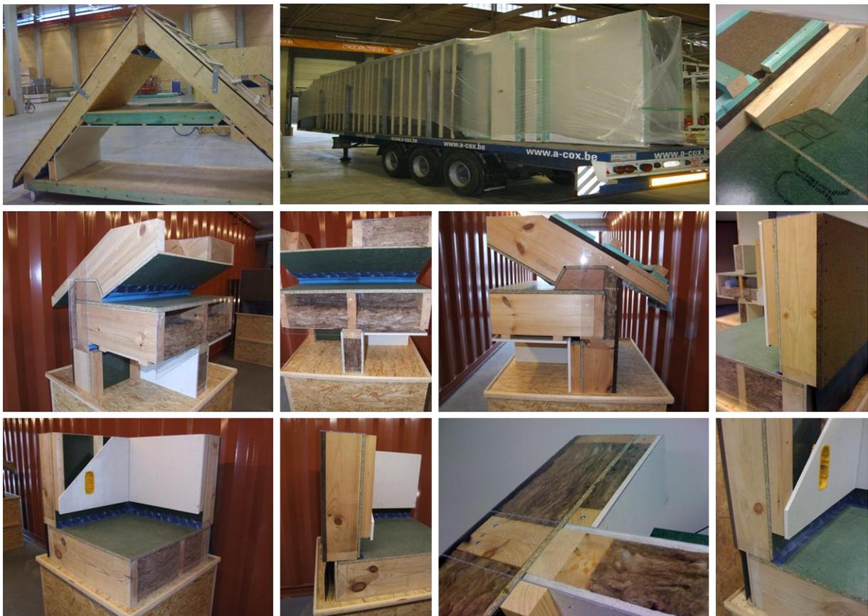
*Figure 2: typical examples of light-weight timber frame constructions and junctions used in free-standing houses. Extending this technology towards terraced houses requires some adaptations but the challenges are huge for building apartment constructions.*
