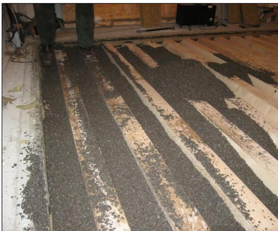
**Floor 'd'** cross laminated timber 9.4 cm thick, with wooden 'ribs' (see drawing) of 9.5x20 cm<sup>2</sup>, interdistance 25 cm. The space between the 'ribs' is filled with gravel (1400 kg/m<sup>3</sup>).
