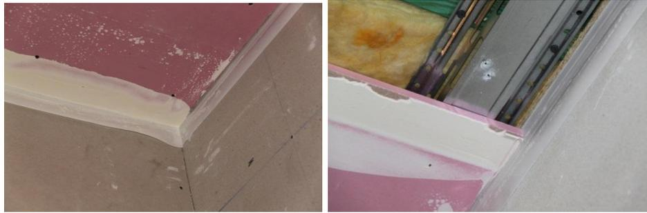
Figure 42 b: creating an elastic joint between the ceiling and the walls can reduce the flanking transmission 'Fd' and 'Df', but can create problems with the fire safety requirements in some countries.
