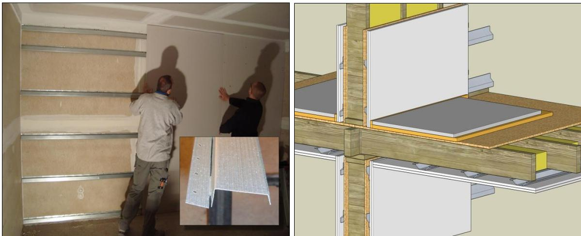
*Figure 42 d: technical linings using resilient studs fixed perpendicular to the wood studs can also diminish some flanking transmission. We do not dispose of any measurements quantifying this, but we expect the improvement to be only in the mid and higher frequencies.*
