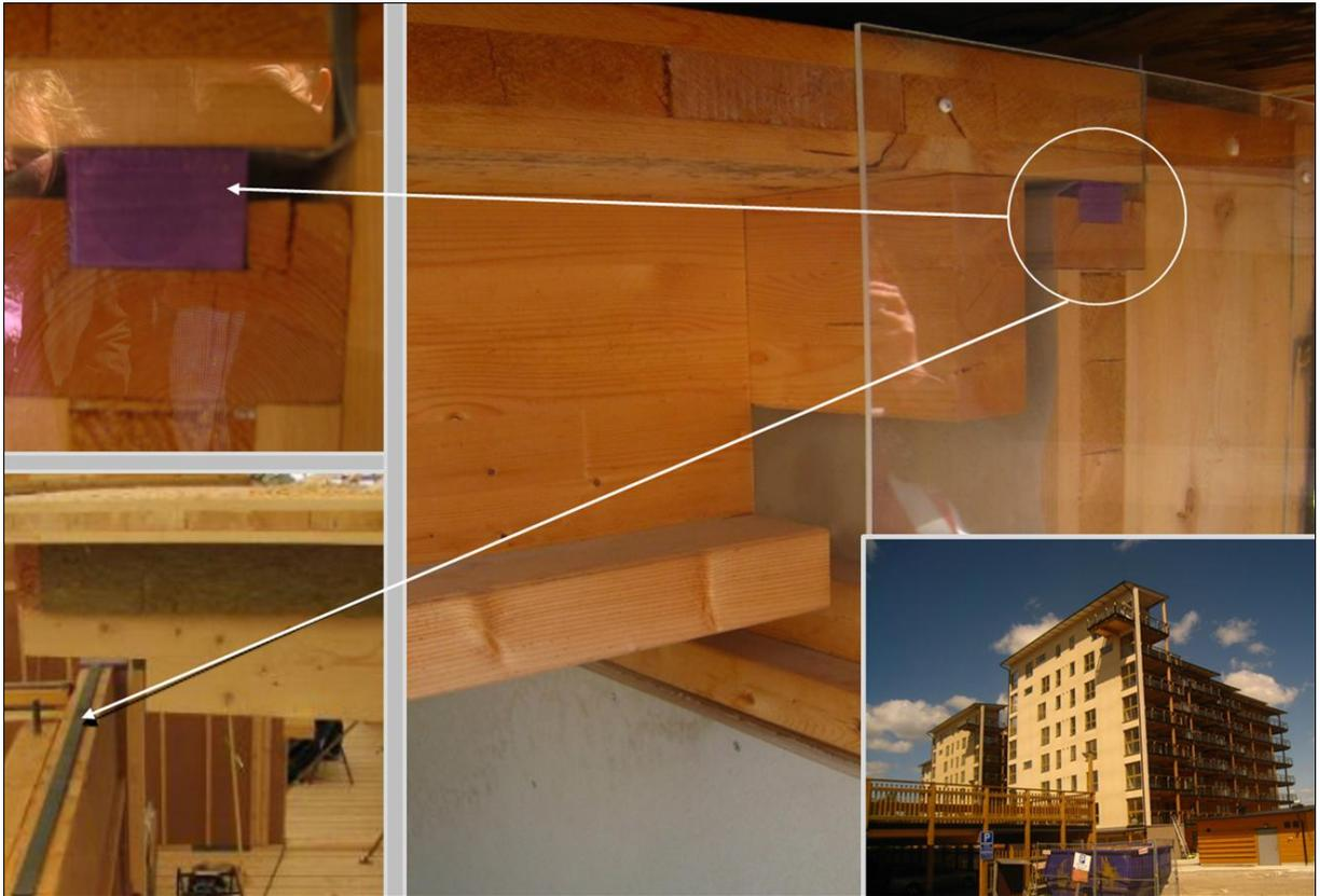
Figure 42 g: a huge multi-storey lightweight timber frame apartment building in Limnologen Växjö, Sweden, also uses linear continuous elastic interlayers to reduce flanking impact sound transmission. All floors bear on the purple elastic interlayer.
