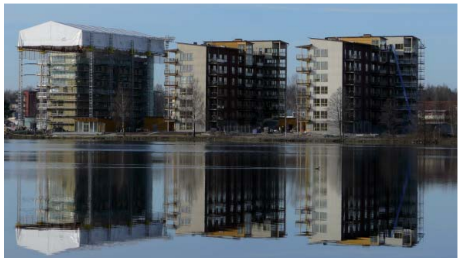
Limnologen in Växjö consists of four 8-storey high residential buildings.
