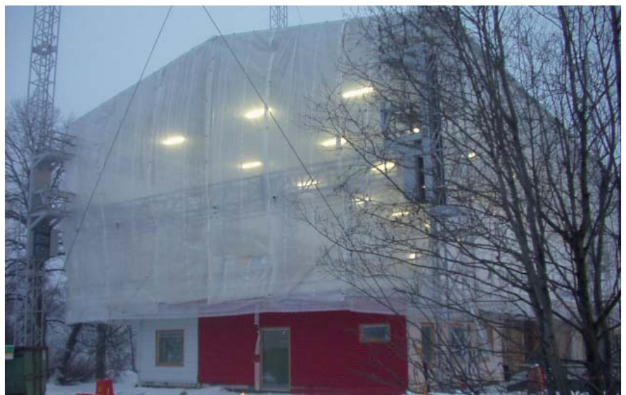
Shelter with assembly platform at Älvsbacka strand in Skellefteå.
