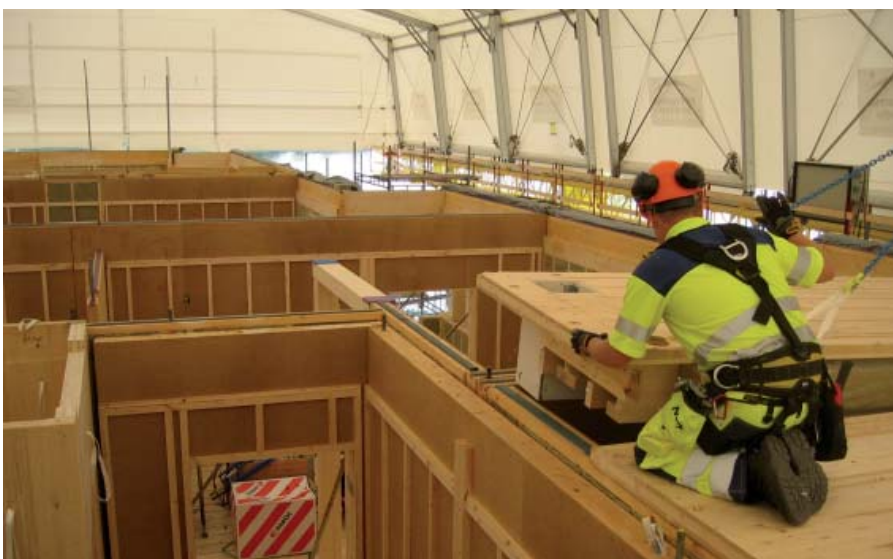
Assembly of floor structures at Limnologen in Växjö.
