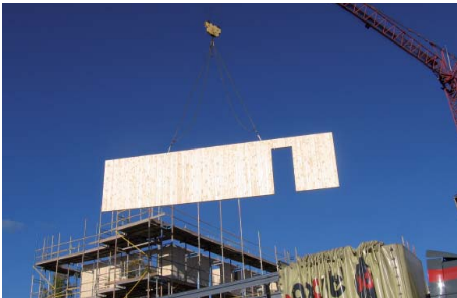
Wall unit on its way at Hyttkammaren in Falun.
