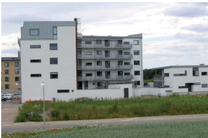
Rydebäck in Helsingborg is a 5-storey residential building.
