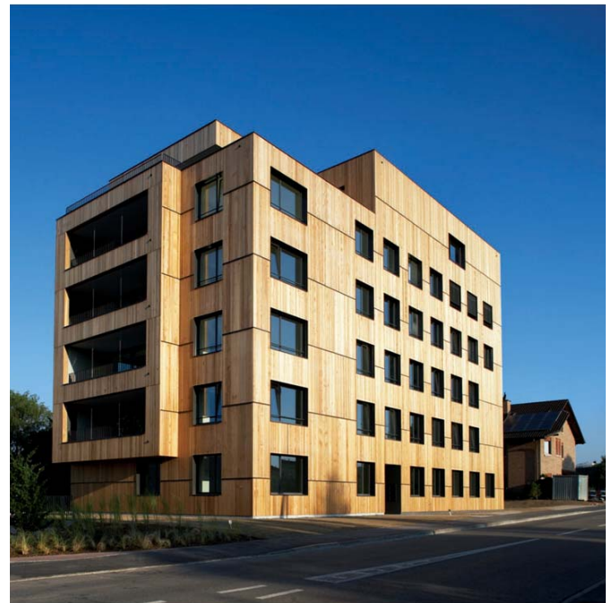
Multifamily house, Zug, Schweiz.
