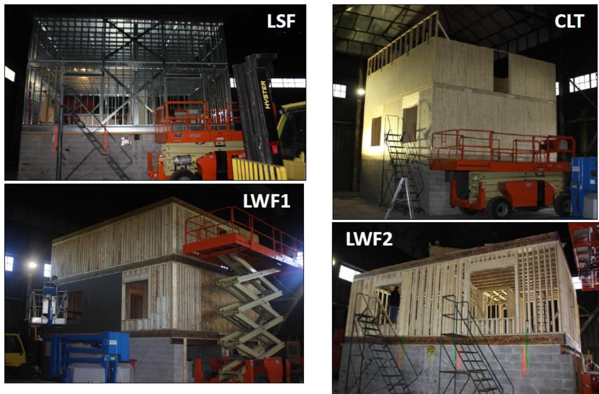
Figure 14: Compartments of test L1 (LWF1), L2 (CLT), L3 (LSF) and L4 (LWF2) under construction, from Su and Lougheed (2014)
