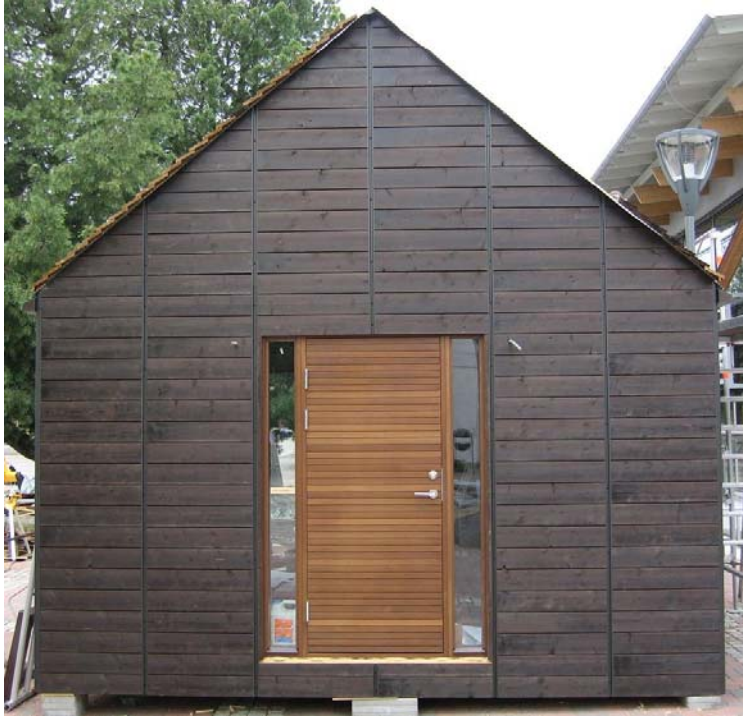
Figure 25: Assembled Cladding
