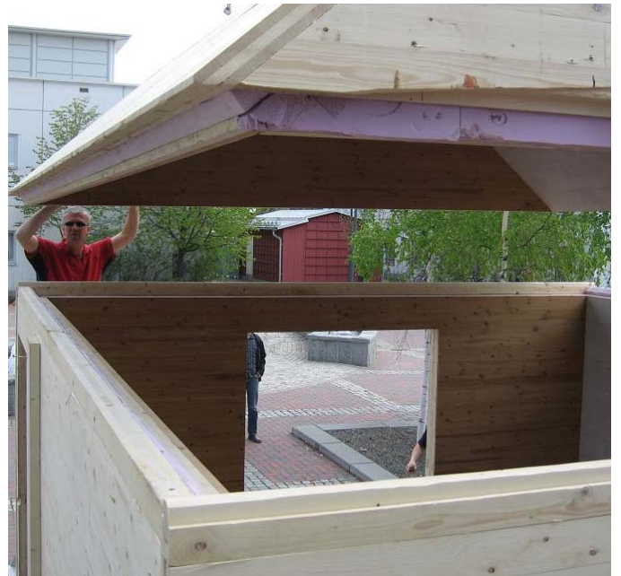
Figure 19: Deliverance of House Frame
