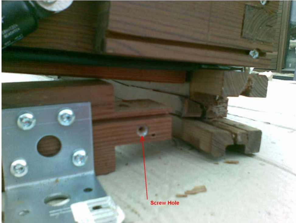
Figure 31: Roof Window Breakage
