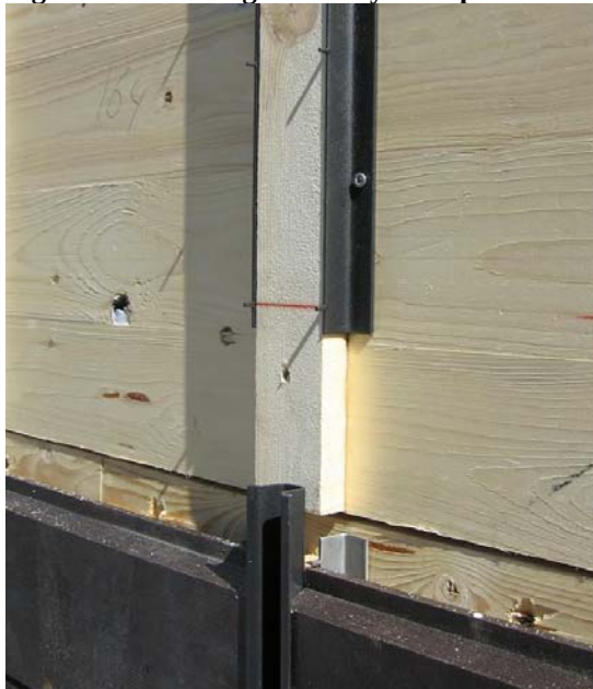
Figure 22: Cladding Assembly Ladder & Clamp
