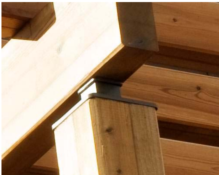
Figure 50: Quadrolite pole Glulam Junction
