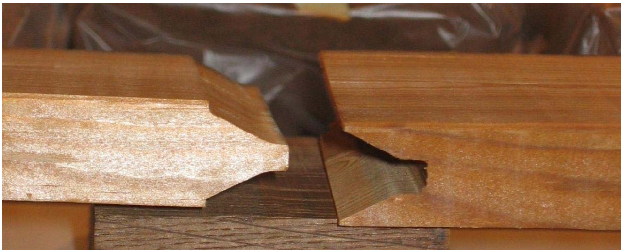
Figure 9: Board Joint Profile for Massive Wood Sheet
