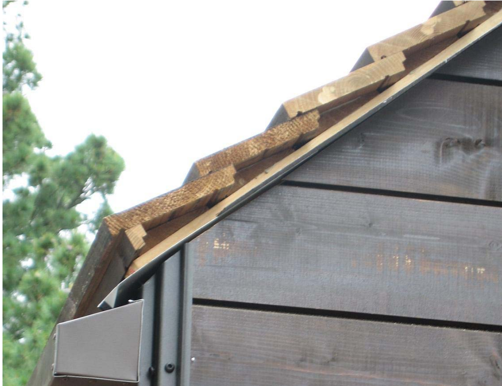
Figure 27: Roof System at Assembling
