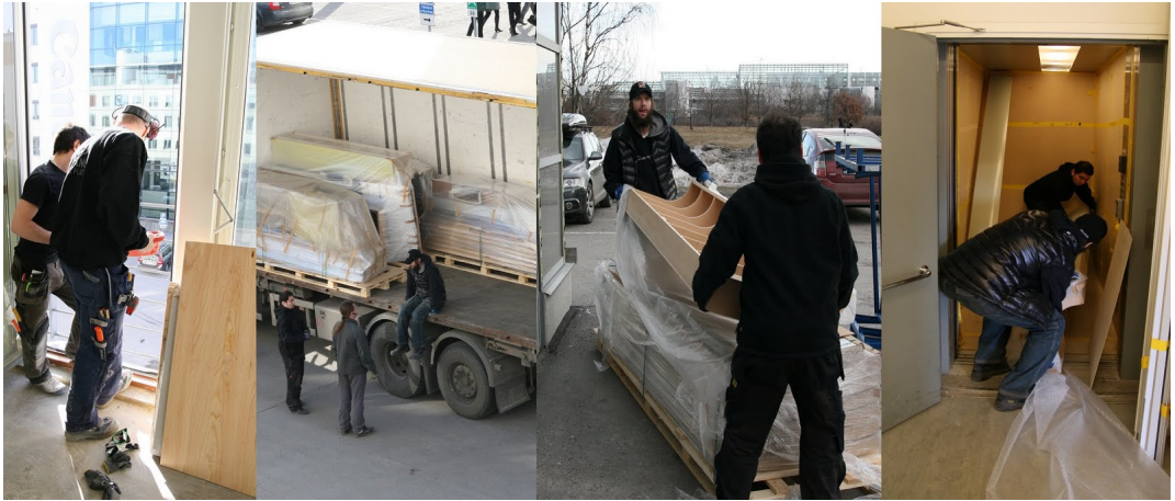
Figure 5: On-site receipt of ETO joinery-product components.
